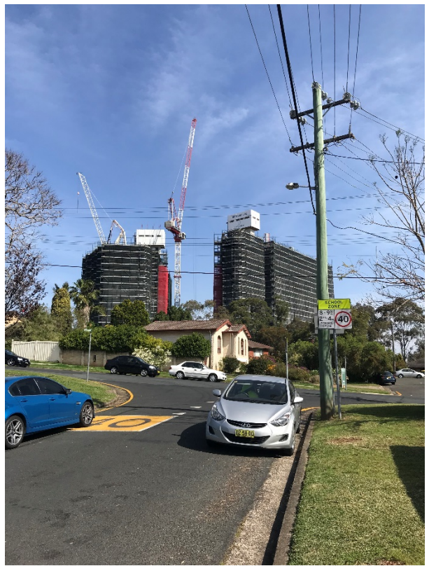
Picture 4 – Looking South Towards Vivien Place From Coolibah Street
